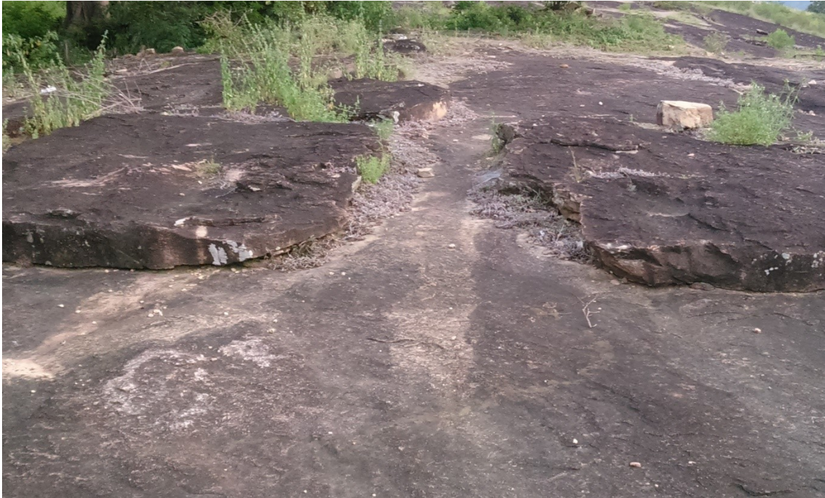
Plate 3. Rock spalling or exfoliation
